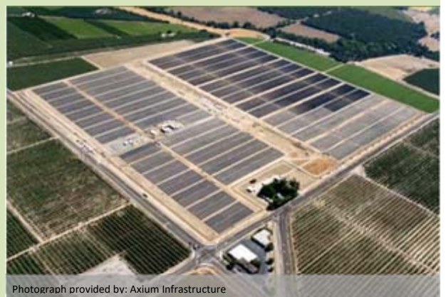
Photograph provided by: Axiom Infrastructure
